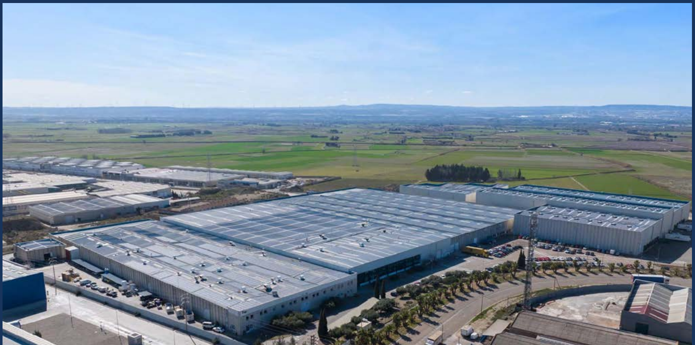
The Malpica 1 property in Zaragoza, Spain was acquired in the third quarter. The property encompasses 63,400 square metres of lettable area and comprises warehouse and industrial premises. The property is fully let.
