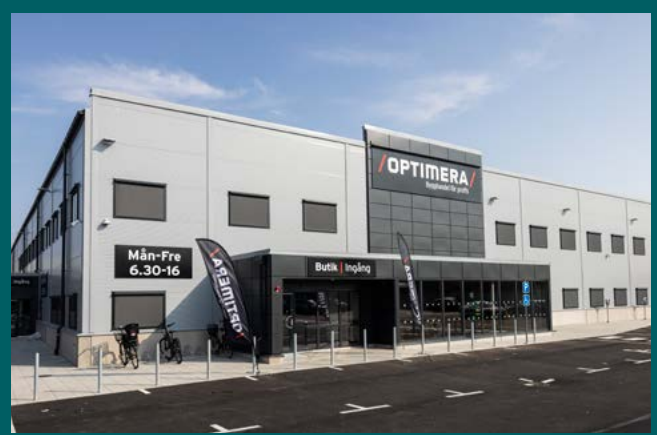
New build on the Bredablick 4 property, Malmö, Sweden. The property has Silver level certification from Miljöbyggnad and is expected to obtain an EPC of B.
