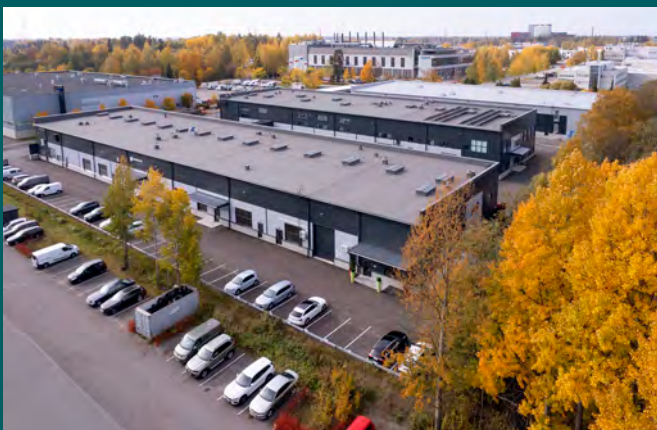
Juurakkotie 5 in Vantaa, outside Helsinki, Finland. The property is certified under BREEAM In-Use Very Good and has an EPC rating of C.
