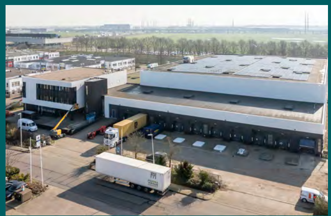
Solar panels at Chroomstraat 140, Zoetermeer, Benelux. The property was certified under BREEAM In-Use Very Good during the year and has an EPC rating of A.
